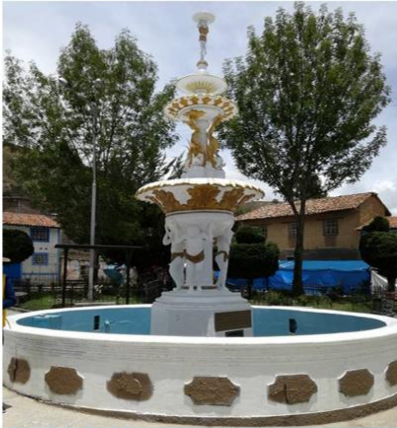
Fig 1. Pileta central restaurada
